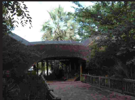
Approach to reception area from courtyard
