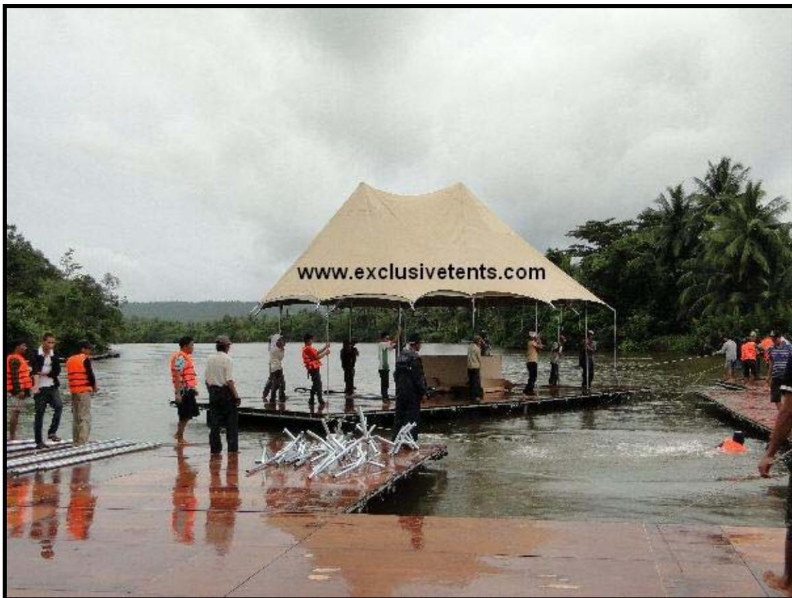
Once on site and despite the rain, the other challenges was setting up the tents on these relatively small flexible floating modules that got overloaded at times with the weight of the tents and all the workers at the same time.
